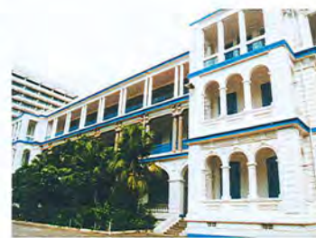
前水警總部近貌。 Recent view of the Former Marine Police Headquarters Compound.
