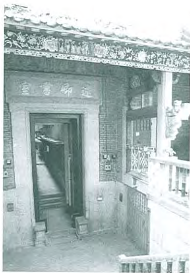
1995年的述卿書室前廳 Entrance Hall of Shut Hing Study Hall, 1995
