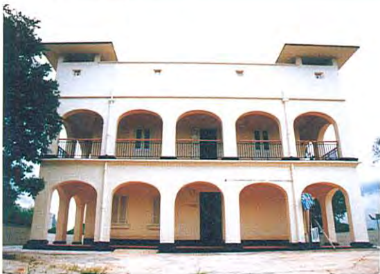
舊屏山警署 Old Ping Shan Police Station
