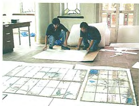
工作人員正在以珍珠棉和塑料中空板包裝玻璃片 The workers were packing the glass panels with polythene foam and polypropylene corrugate board
