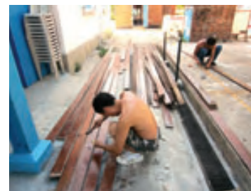
維修木地板 Repairing of timber board
