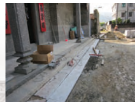
用麻石重鋪前院以改善地面的排水情況 Repaved forecourt with granite slabs allowing for surface run-off
