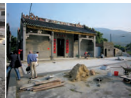
用麻石重鋪前院以改善地面的排水情況 Repaved forecourt with granite slabs allowing for surface run-off
