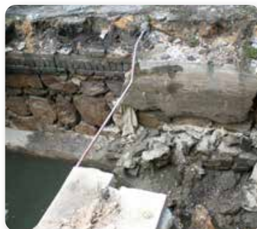
不穩固的花崗石護土牆結構 Unstable structure of the granite retaining wall
