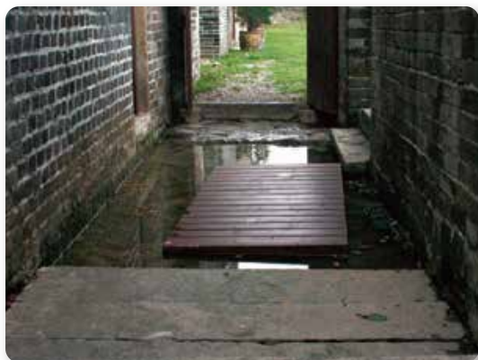
改善工程展開前，戶外走廊曾出現水浸問題。 Flooding at the external corridor before the improvement works
