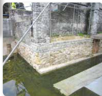
加固後的花崗石護土牆 Granite retaining wall after consolidation
