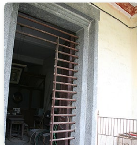
正門的金屬趟櫳門 Metal sliding door at the main entrance
