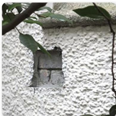
採集外牆樣本 A field sample is cored out from an external wall.
