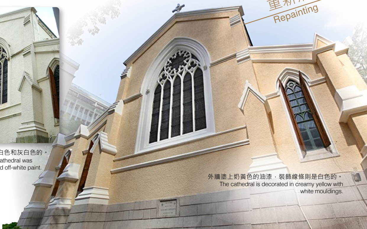
以原有的物料來修復外牆批盪 Application of the rendering mix matched with the existing materials
