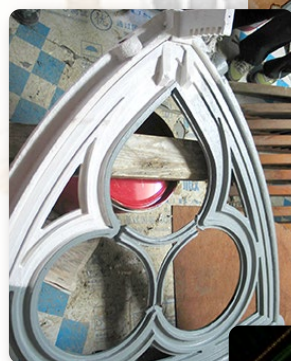
修復和重置鑄鐵窗 Repair and Reinstatement of the cast iron window
