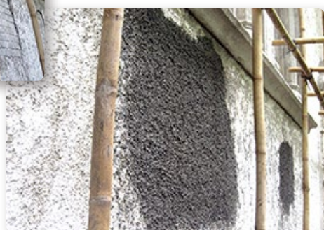
以原有的物料來修復外牆批盪 Application of the rendering mix matched with the existing materials
