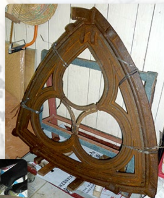
修復和重置鑄鐵窗 Repair and Reinstatement of the cast iron window
