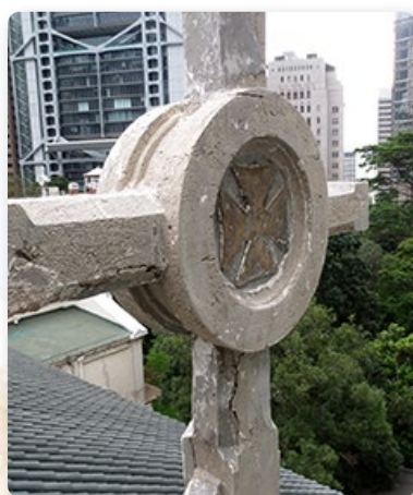
十字架裝飾的裂痕 Cross finial with cracks
