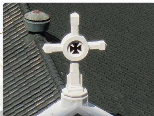
復修後的十字架裝飾 The cross finial after repair
