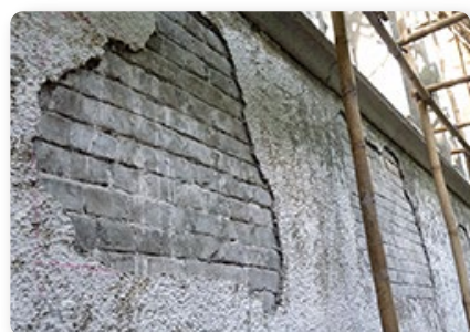
水泥混合碎石批盪脫落 The deboned roughcast rendering
