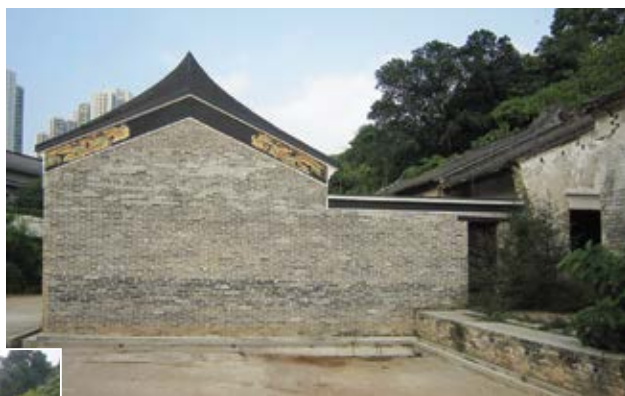
地面回復原來高度，填土痕跡清晰可見。 The land was excavated back to its original level; the mark left by the previous land filling can clearly be seen.
