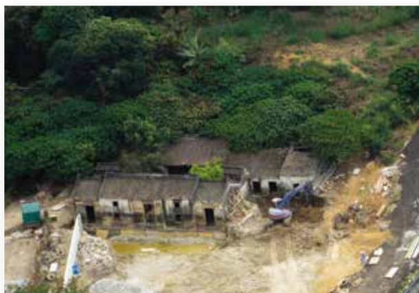
達德公所周圍被填高，天然排水系統受破壞，工程把填土移走。 The surrounding areas of Tat Tak Communal Hall were filled in and the natural drainage system was blocked. Soil and debris were removed during the works.
