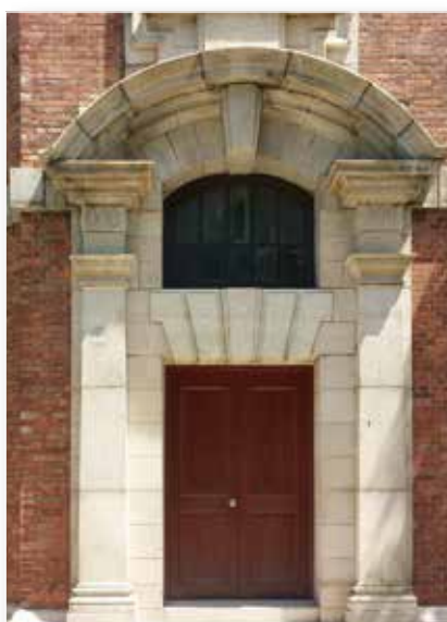
用扇形拱窗、楣飾、拱頂石及壁柱裝飾的入口 Decorative entrance with segmental arch, pediment, keystone and pilasters
