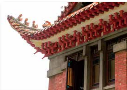
琉璃瓦頂及其飛檐、斗拱和陶塑蹲獸 Glazed tile roof with flying eaves, brackets and ceramic running animals
