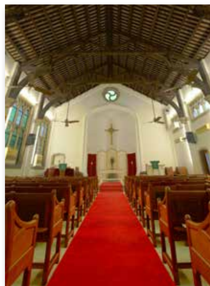
由兩組托臂樑支撐的中式金字瓦頂 A Chinese-tiled pitched roof is supported by double hammer-beam timber roof trusses
