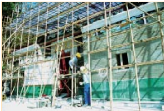
▲ 維修工人把古廟後期加建及不協調的部分清除，回復建築物本來面貌 Craftsmen removing inappropriate repairs and additions conducted in previous renovations to restore the temple's original appearance
