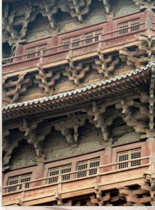
有「百尺蓮開」美喻的木塔斗栱結構 The dougong construction of interlocking wooden brackets of the pagoda is given the enchanting name, "A Hundred Blossoming Lotuses"
