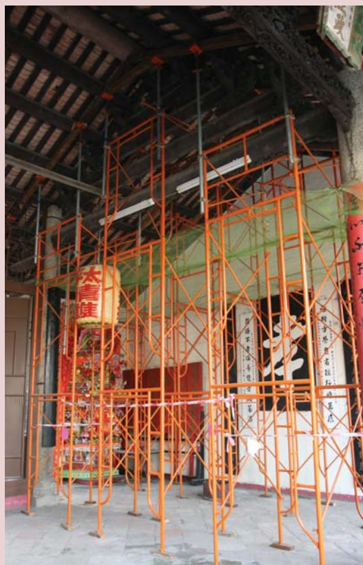
▲ 臨時撐架為宗祠鞏固天面結構 Temporary metal frames erected to support the timber roof structures
