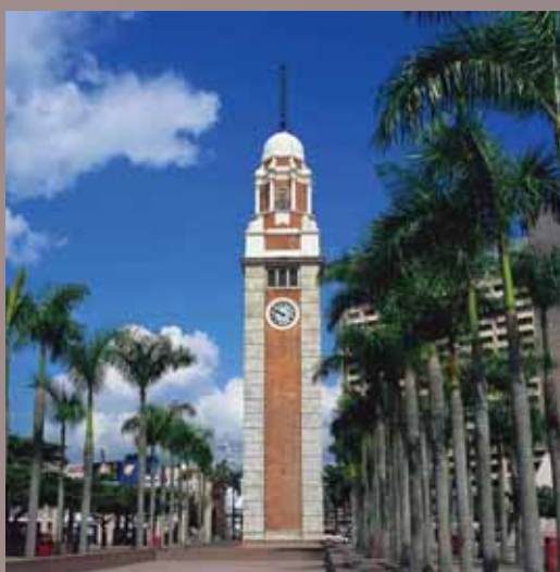
鐘樓採用新古典風格設計，樓高44米，以紅磚和花崗岩建成 The Clock Tower with Neo-Classical design is 44m tall, built with red bricks and granite blocks
