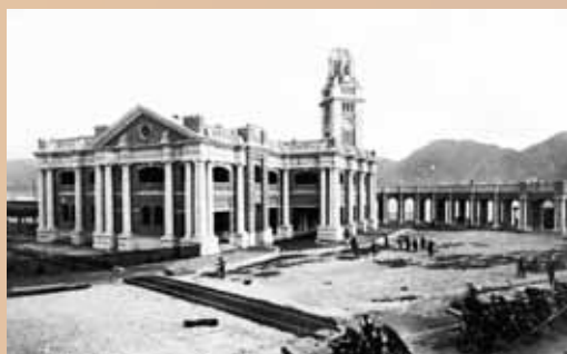
火車總站大樓興建工程進入最後階段 The terminal building in the final stage of construction
