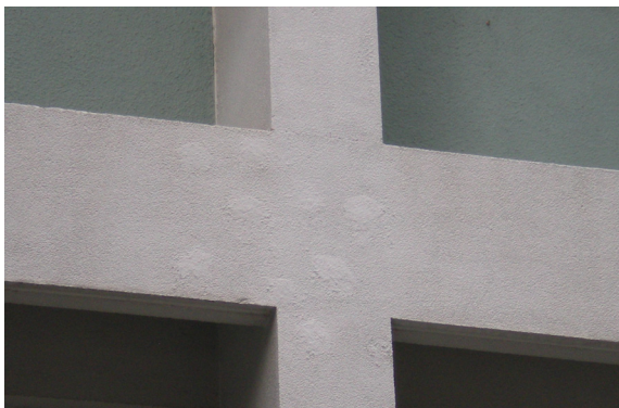
Concrete repairs on the West Wing
