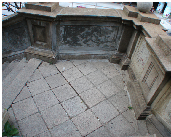
Concrete repairs and gaps in the paving of the Battery Path steps
