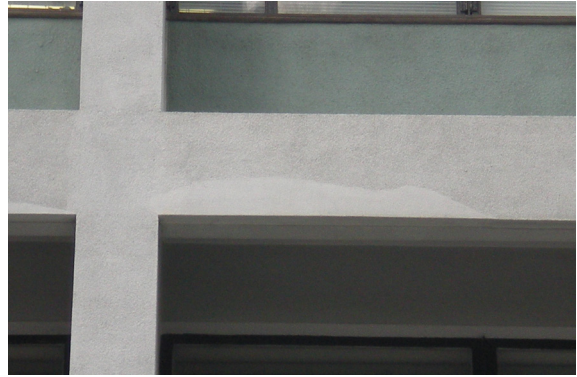
Concrete repairs to arrisses
