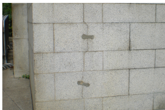
Cracks in the granite walling
