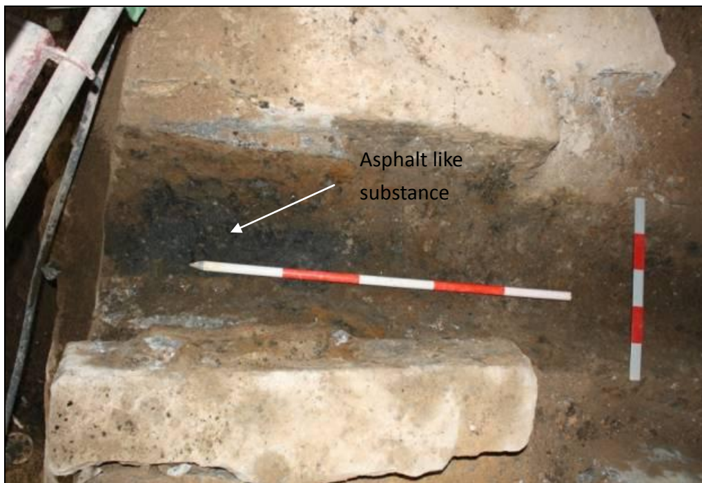
Plate 8c Inside of stone drain, notice black asphalt substance inside
