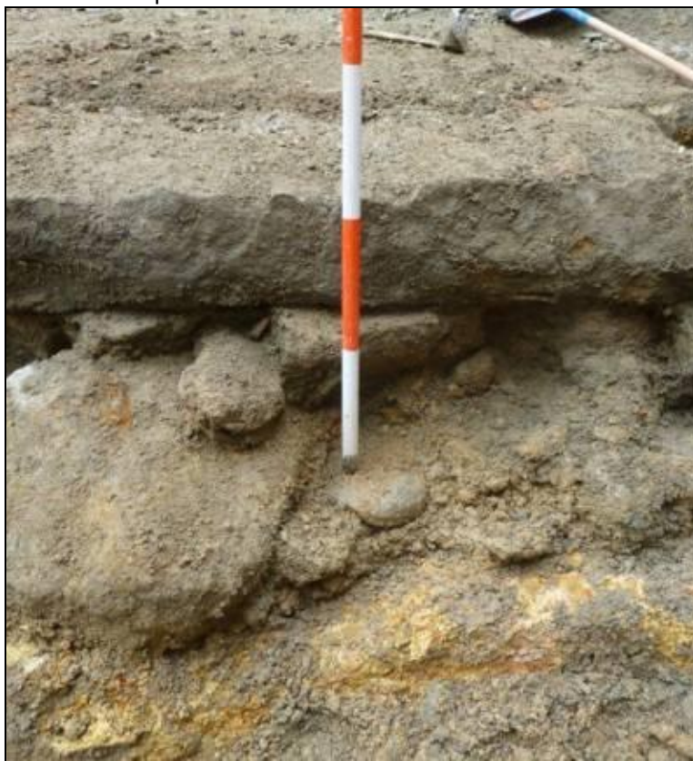
Plate 12c Seawall foundation (context 206): use of natural stones in foundation
