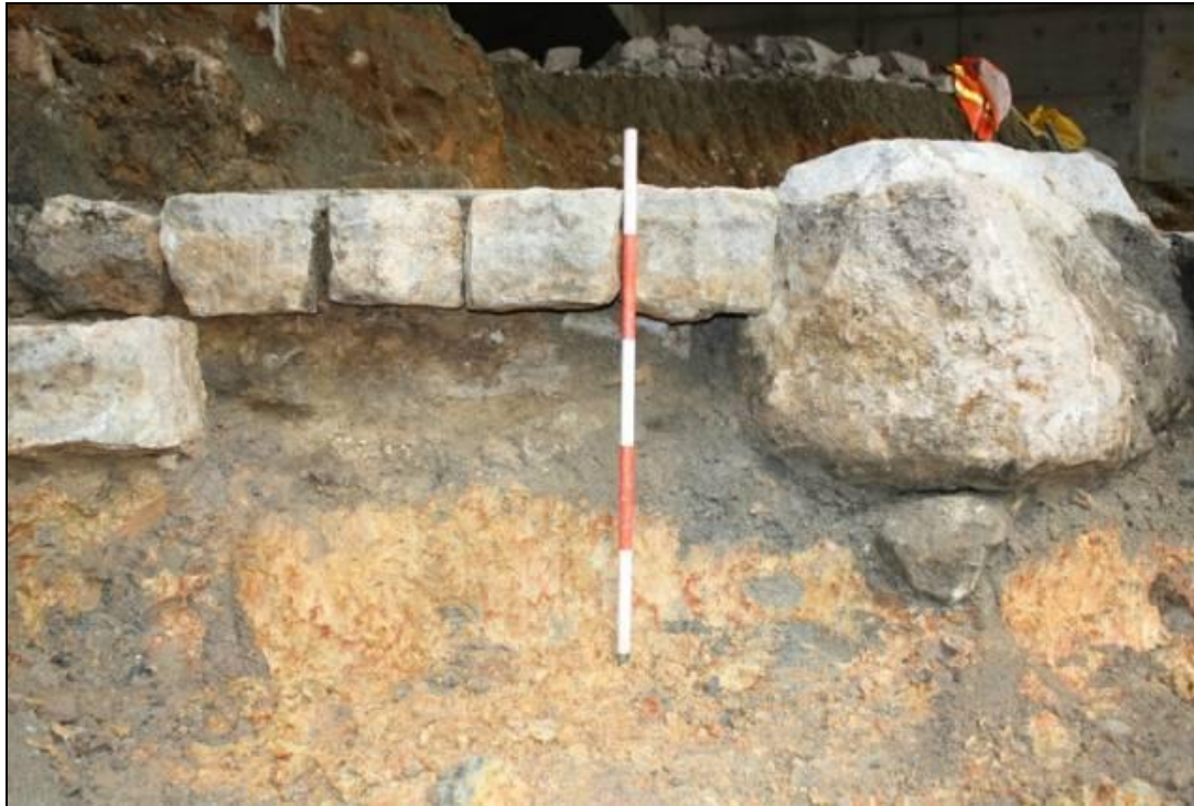
Plate 12d Seawall foundation: missing foundation blocks near and under stone drain, context 210
