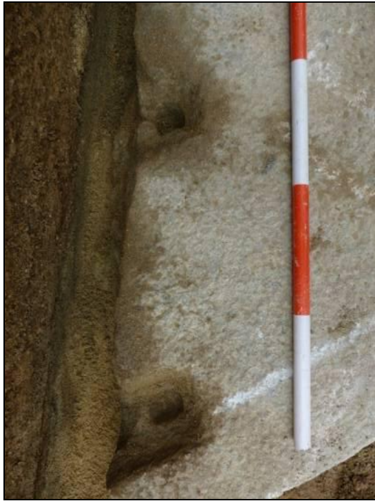
Plate 11d Detail of the 'lewis' holes
