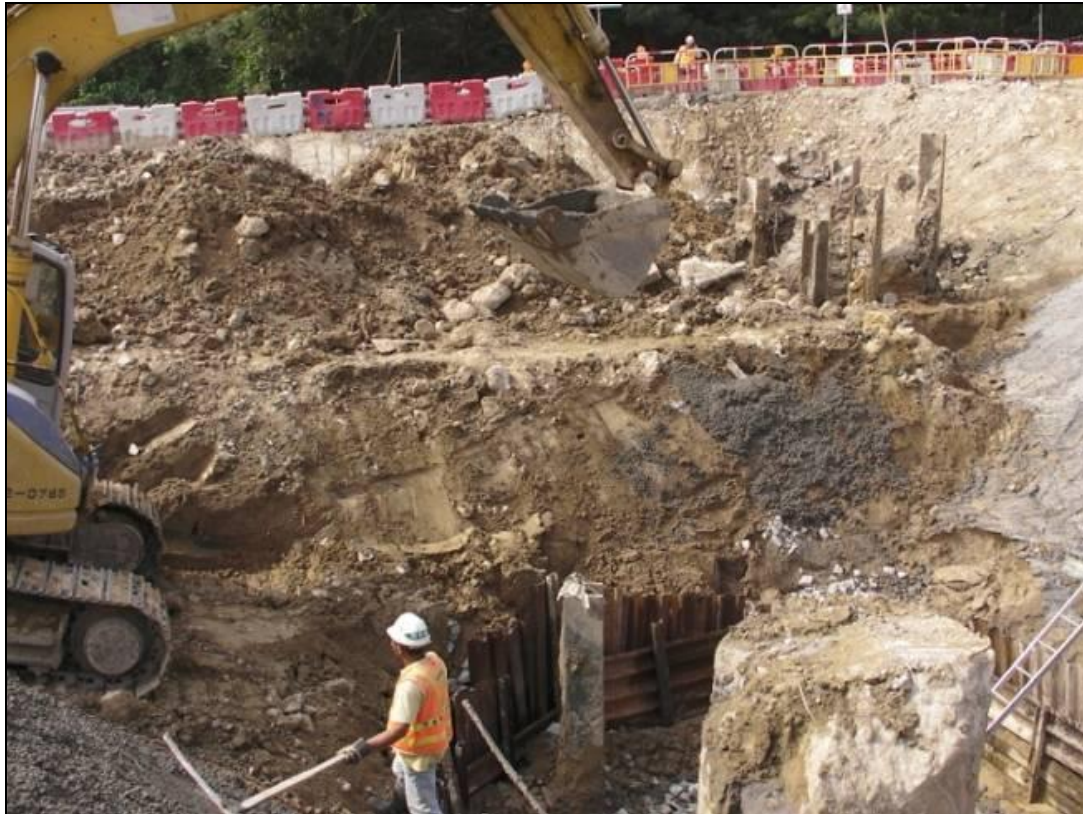
Plate 15 Sheet piling of previous development at base of hill slope
