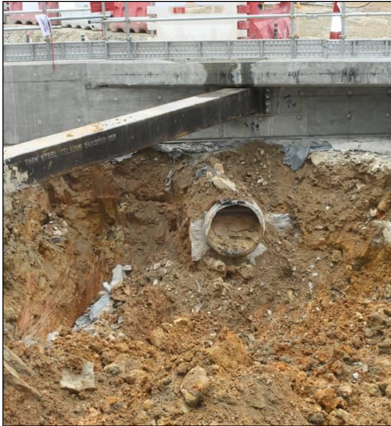
Plate 5 Modern concrete pipe noticed within SEE Shaft and which cut top of well shaft
