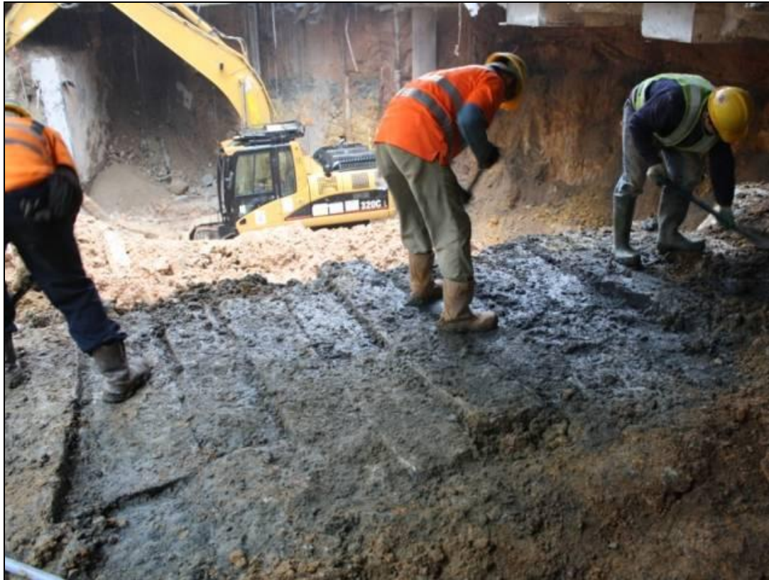
Plate 12b Seawall foundation: cleaning of top of foundation Part 'B' (context 206); some blocks span the width of the foundation
