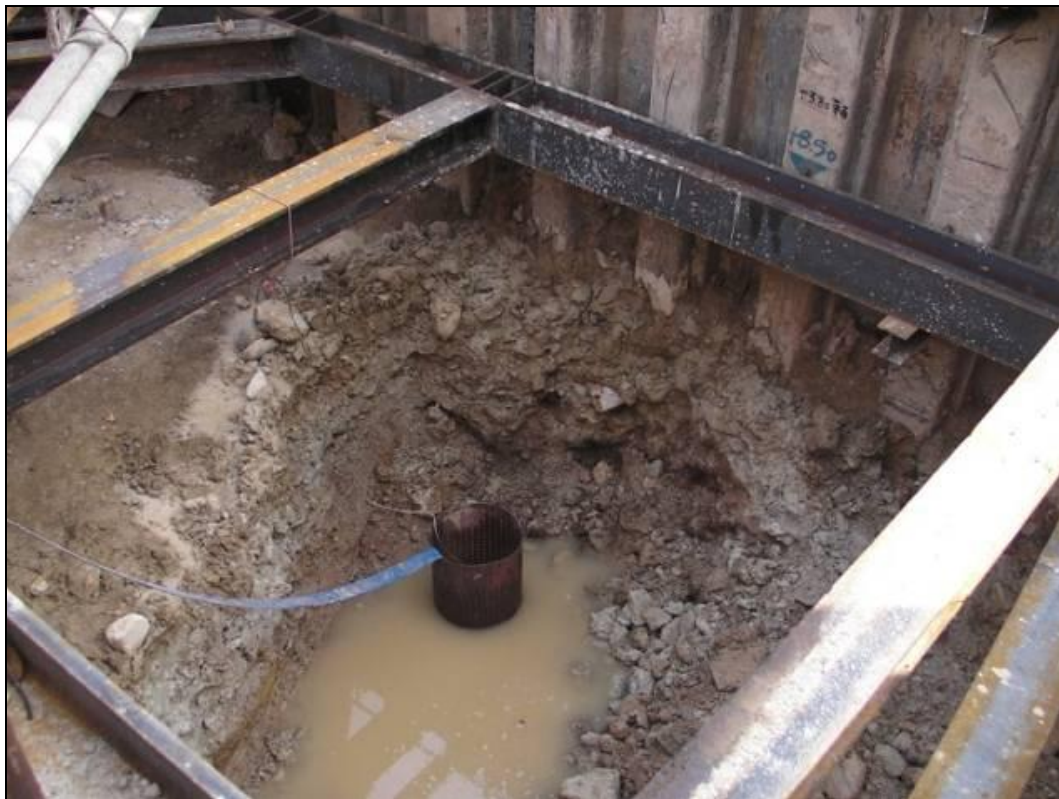
Plate 17b View of pile cap excavations at Site 10, Pier B4, looking north-northwest
