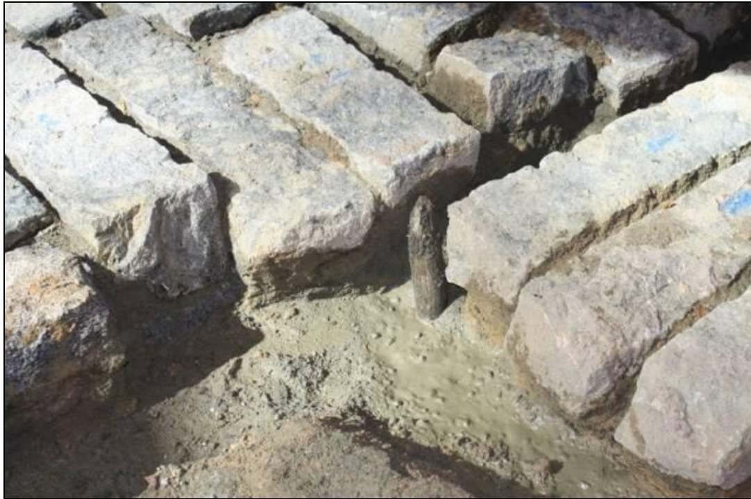
Plate 12f Seawall foundation: wooden post noticed at rear of foundation near buttress
