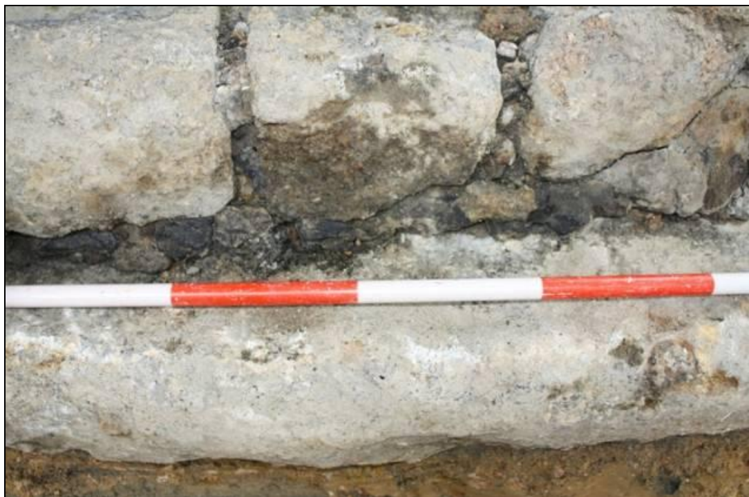
Plate 12i Seawall foundation: deteriorated grouting used at foundation
