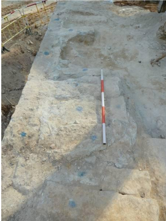
Area of concrete on top of surviving seawall fragment
