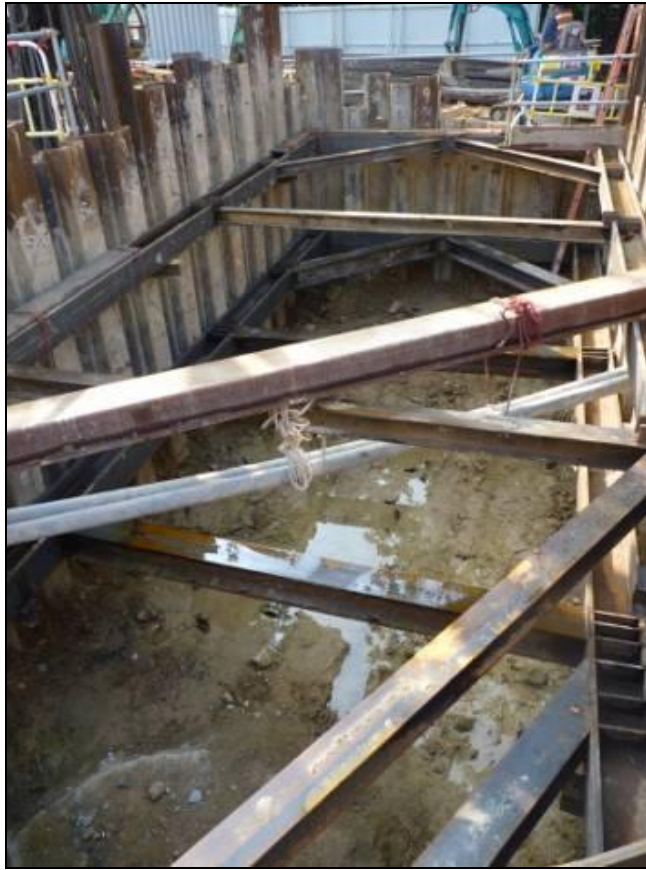
Plate 17a View of pile cap excavations at Site 10, Pier B4, looking west
