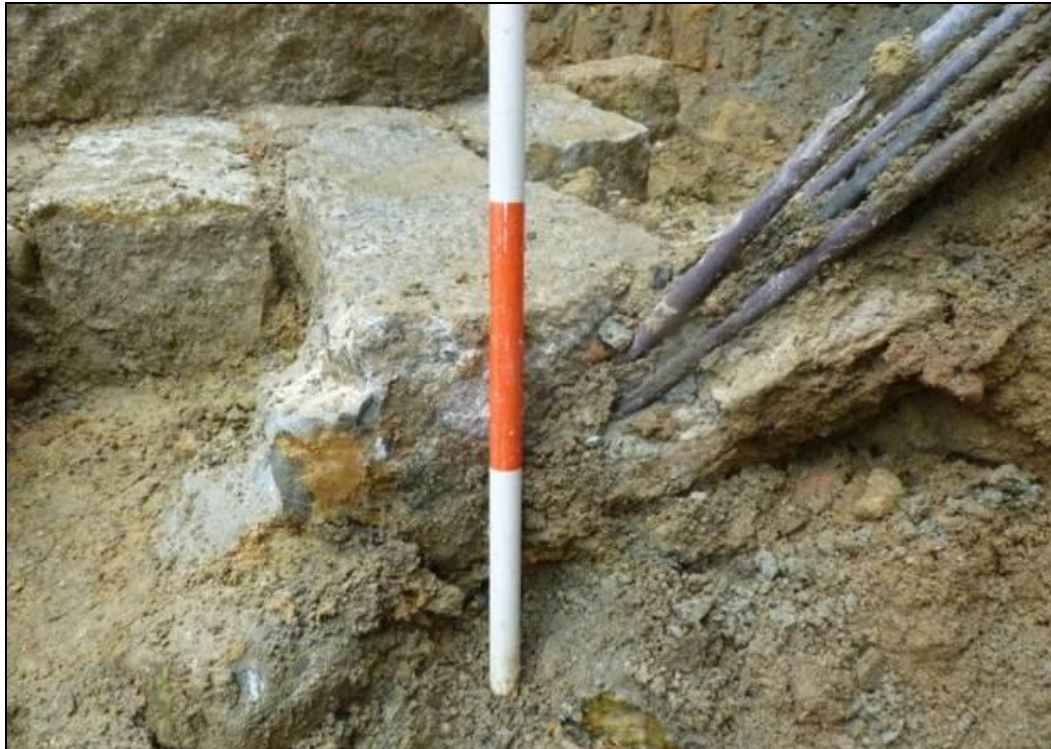
Plate 13a Damaged seawall foundation: metal brace and sheet piling associated with former Admiralty Station Entrance 'E' which disturbed the foundation at the western end
