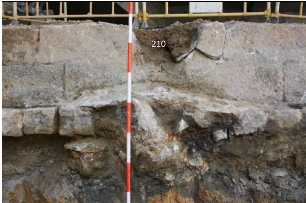
Plate 8b Bottom of stone drain with replaced concrete foundation and natural stone
