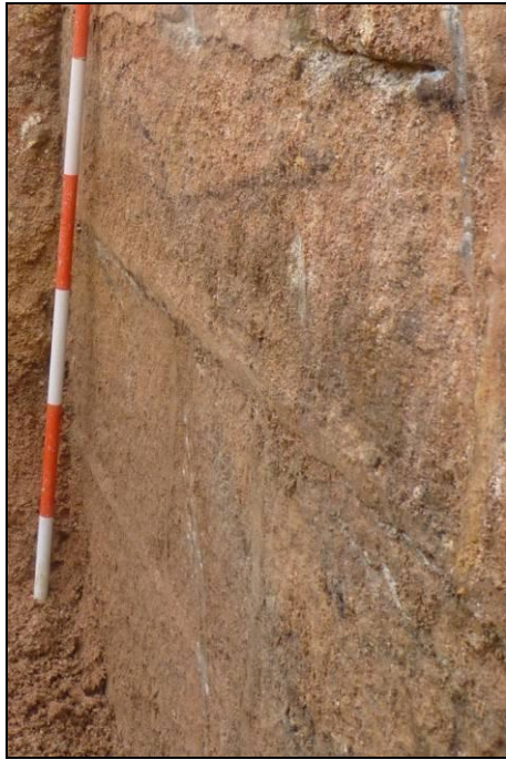
Plate 7 Sealing of cracks between dressed granite façade blocks
