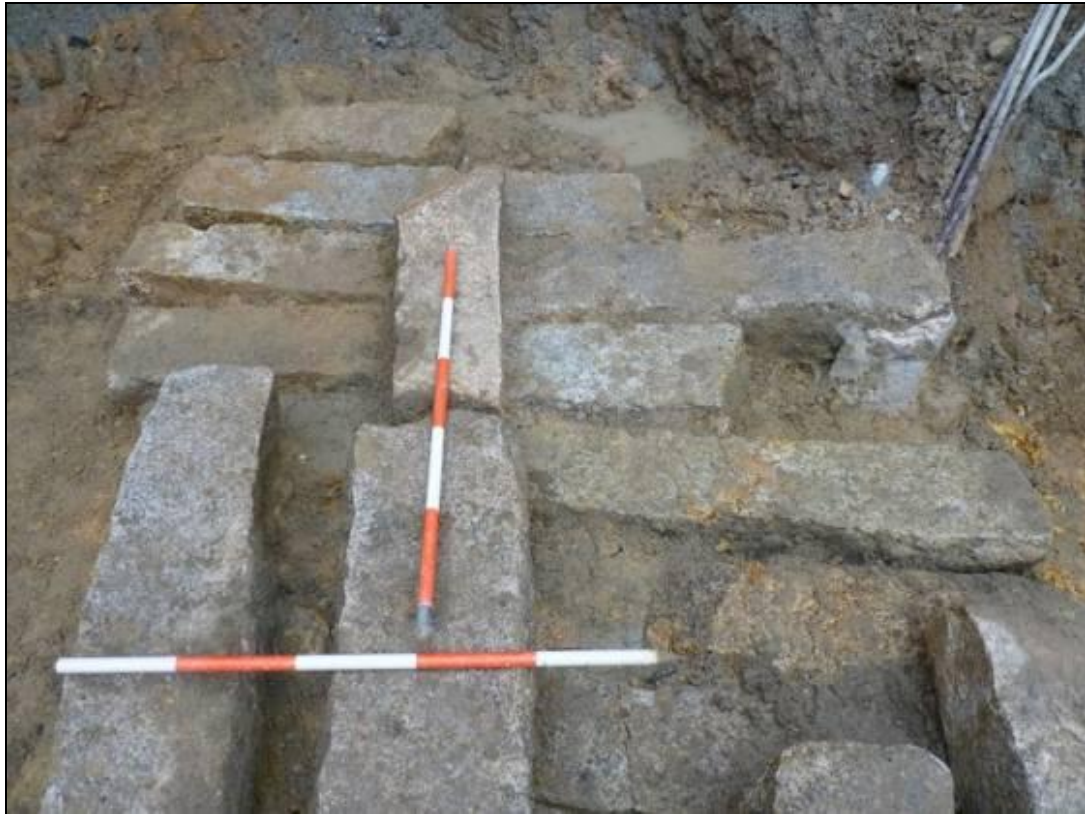
Plate 12j Seawall foundation: a simple bond
