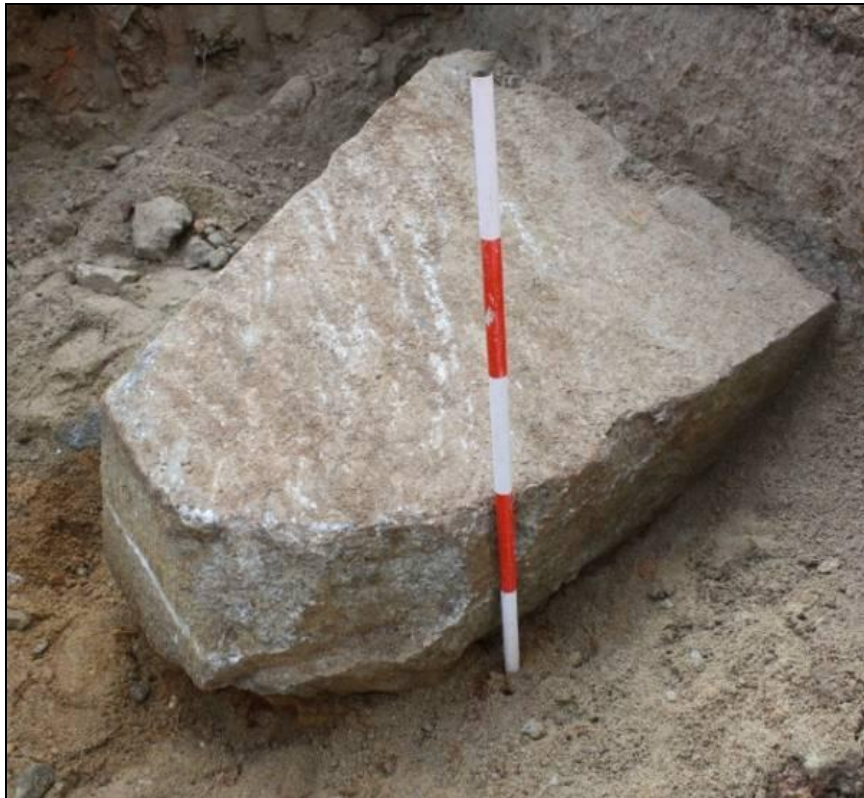
Plate 11c Landing stone immediately in front of the seawall; notice the 'lewis' holes against the seawall and thickness of stone
