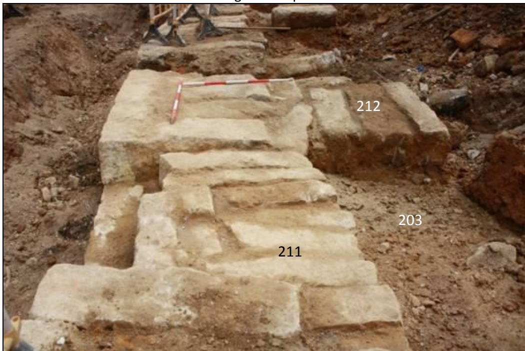
Plate 6f View of the seawall fragment: detail view of buttress backing the south of the seawall
