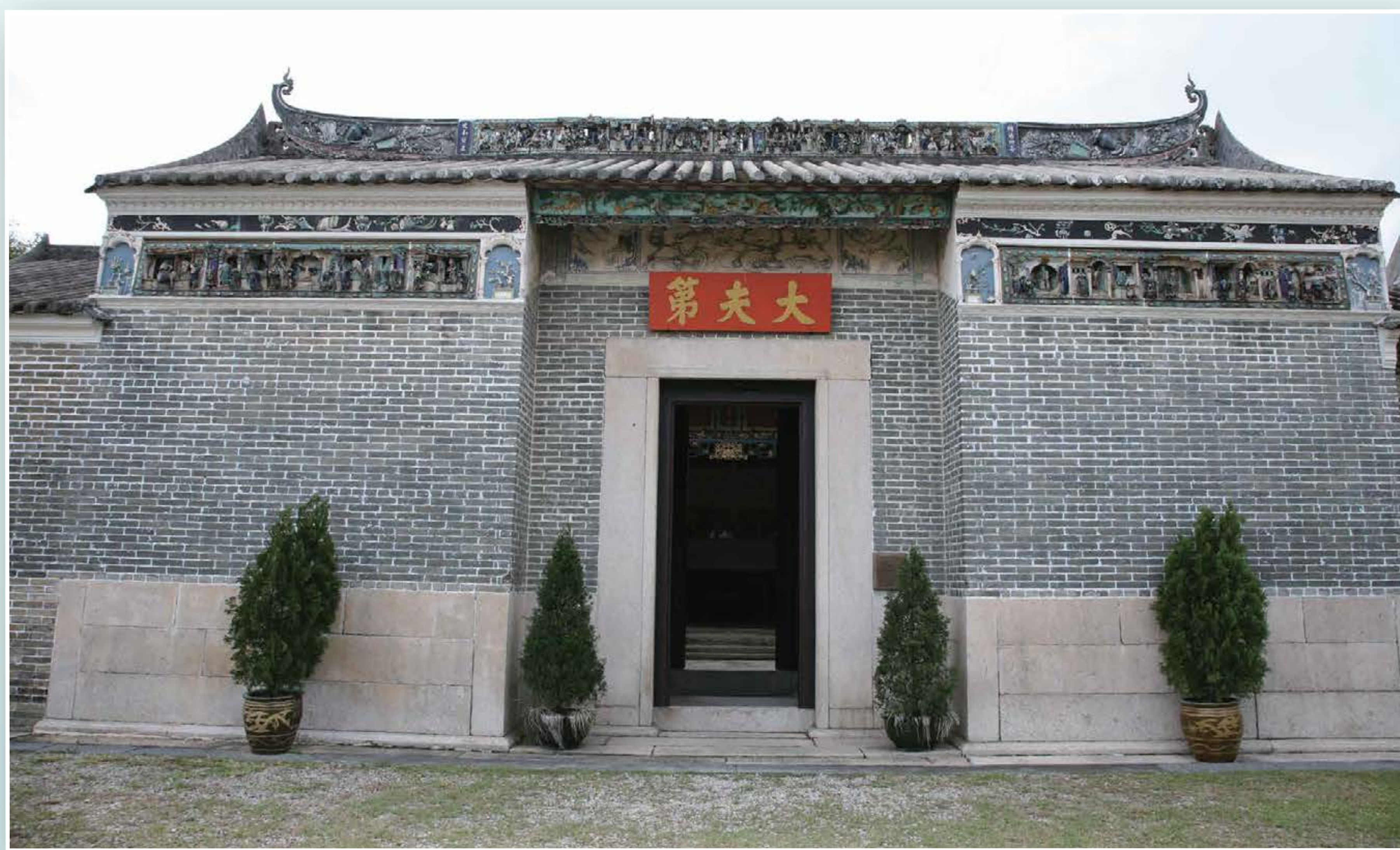
修復後的外貌 Facade after restoration
