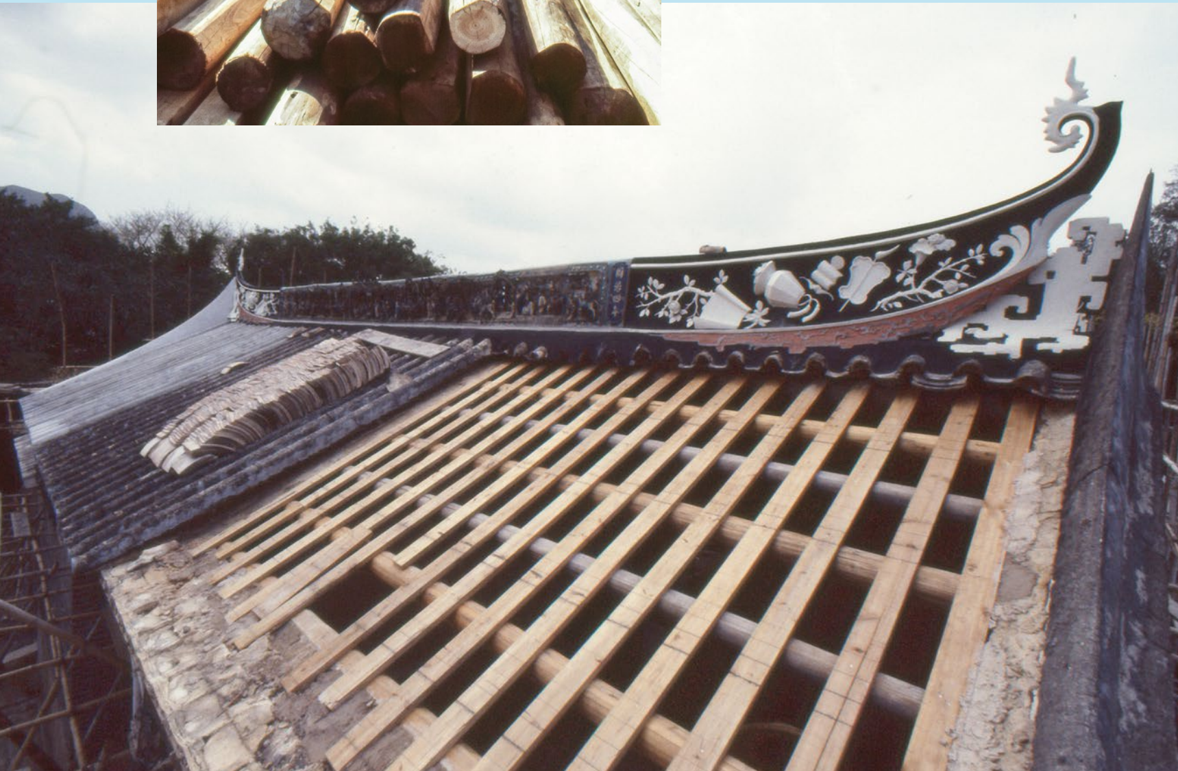
鋪砌天面瓦頂 Laying of roof tiles
