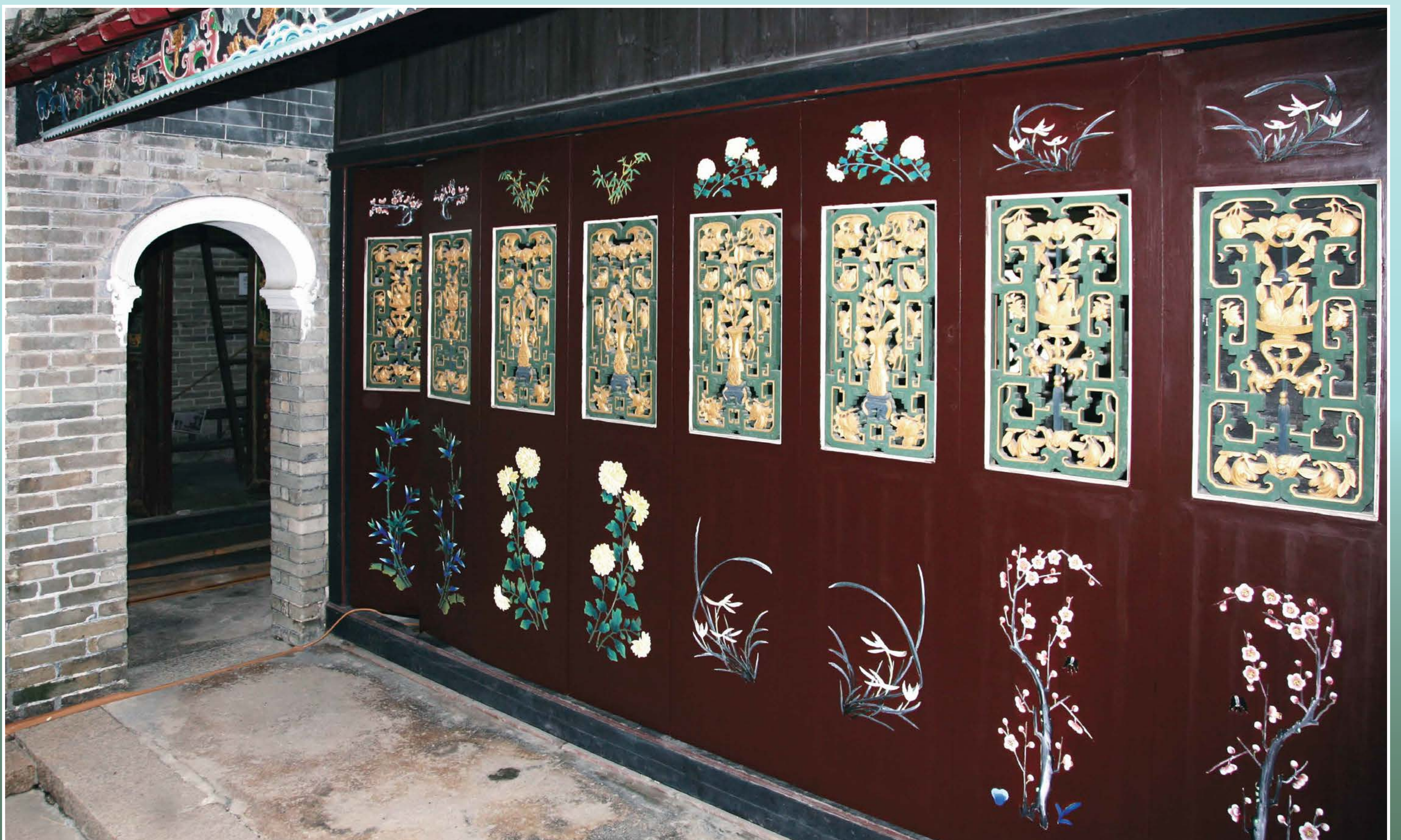
重修後的木屏風 Carved wooden panels after restoration
