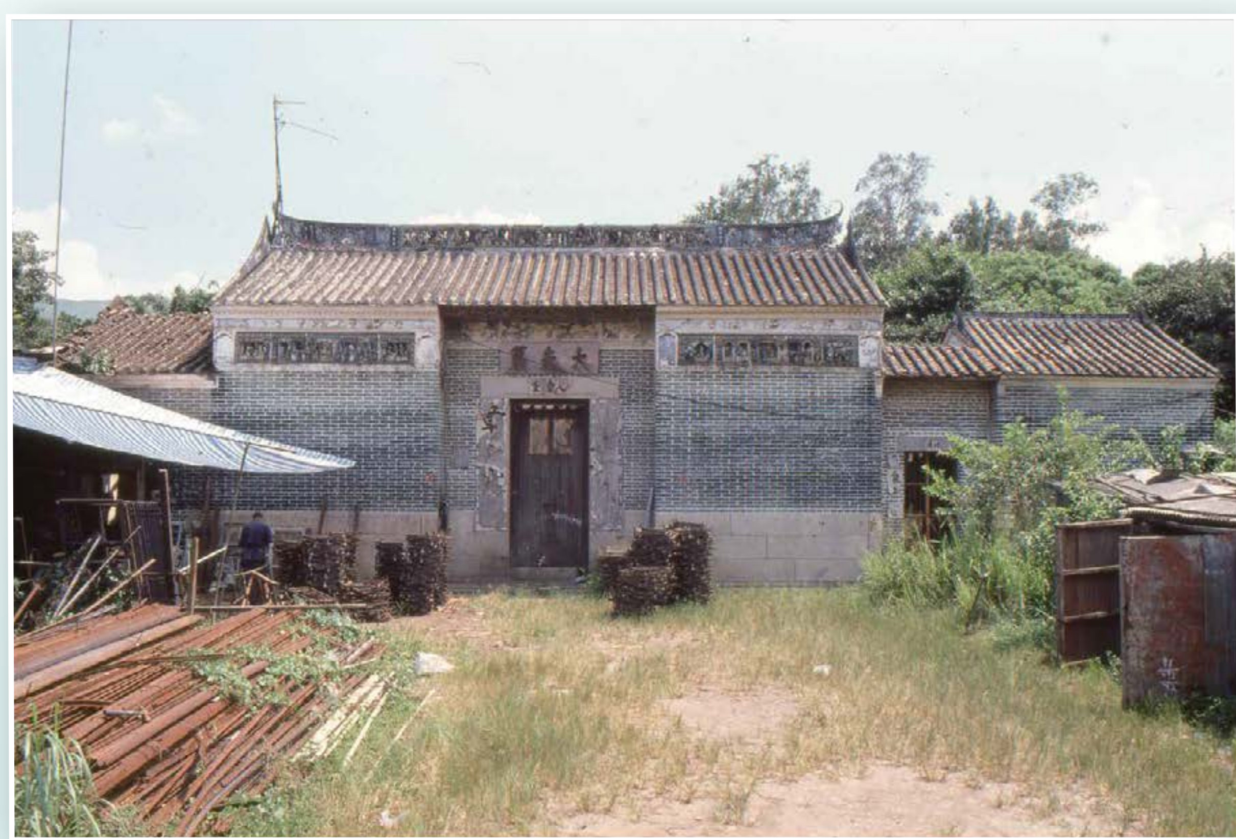
修復前的外貌 Facade before restoration
