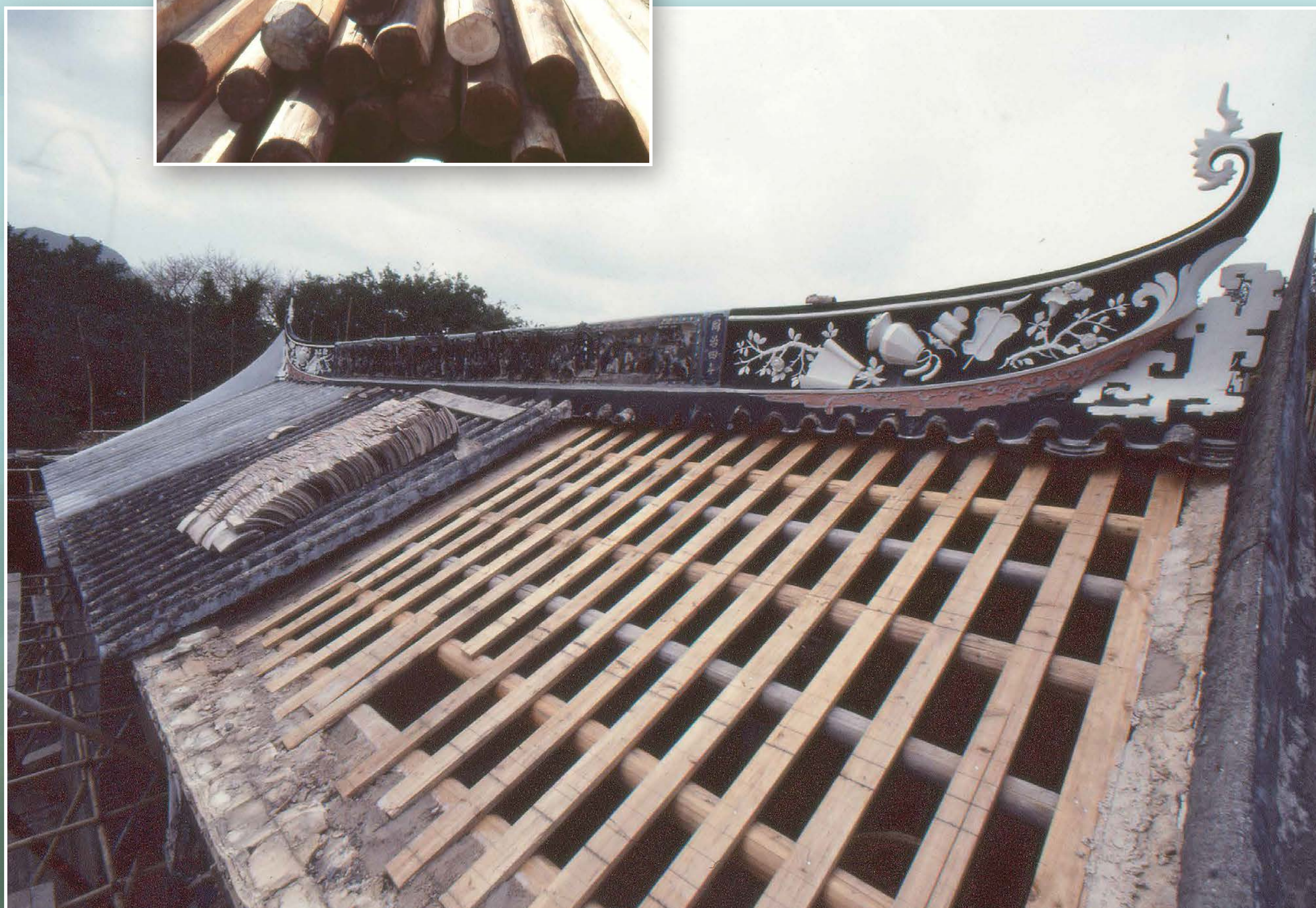
鋪砌天面瓦頂 Laying of roof tiles
