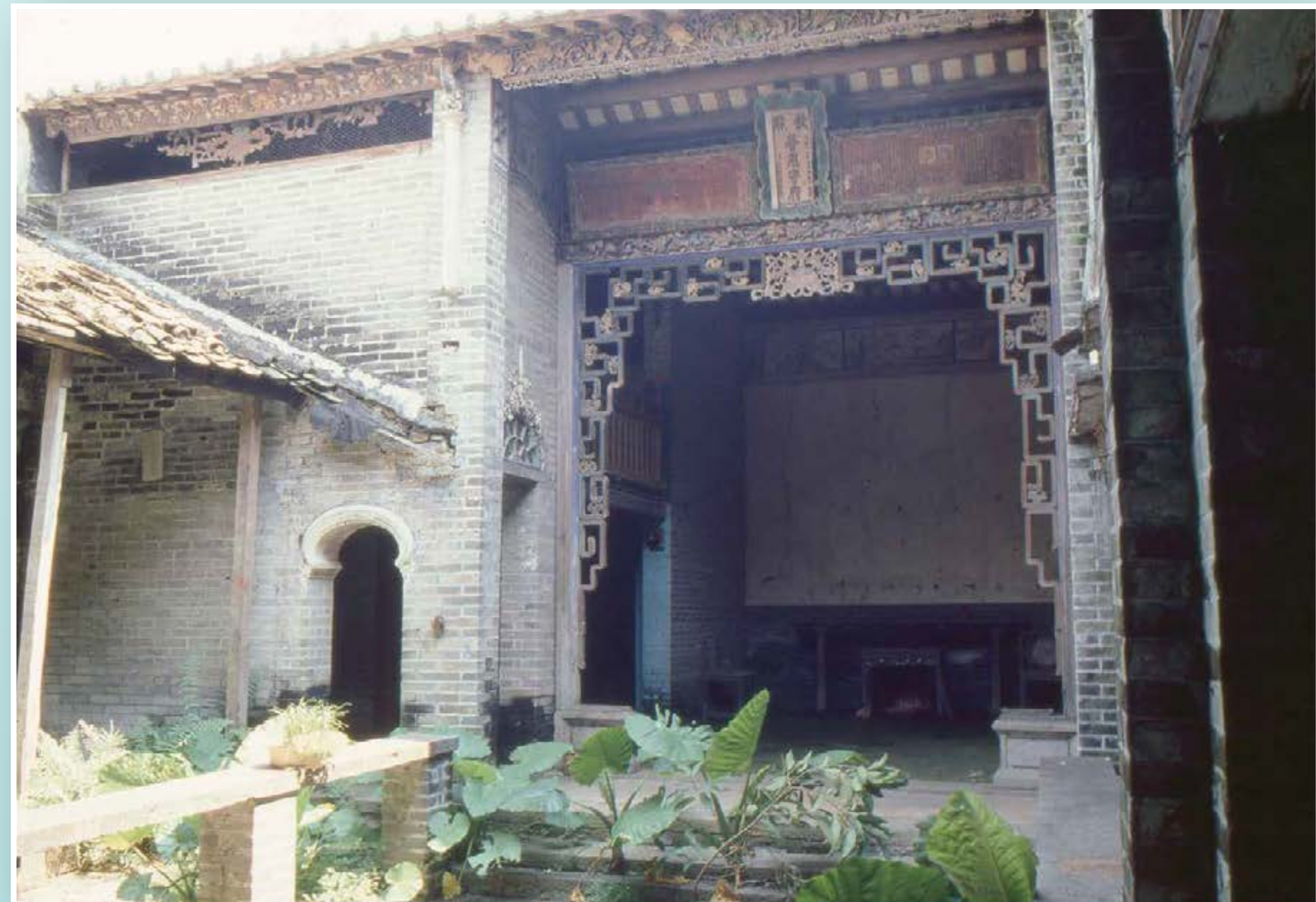
修復前的內貌 Interior view of the building before restoration
