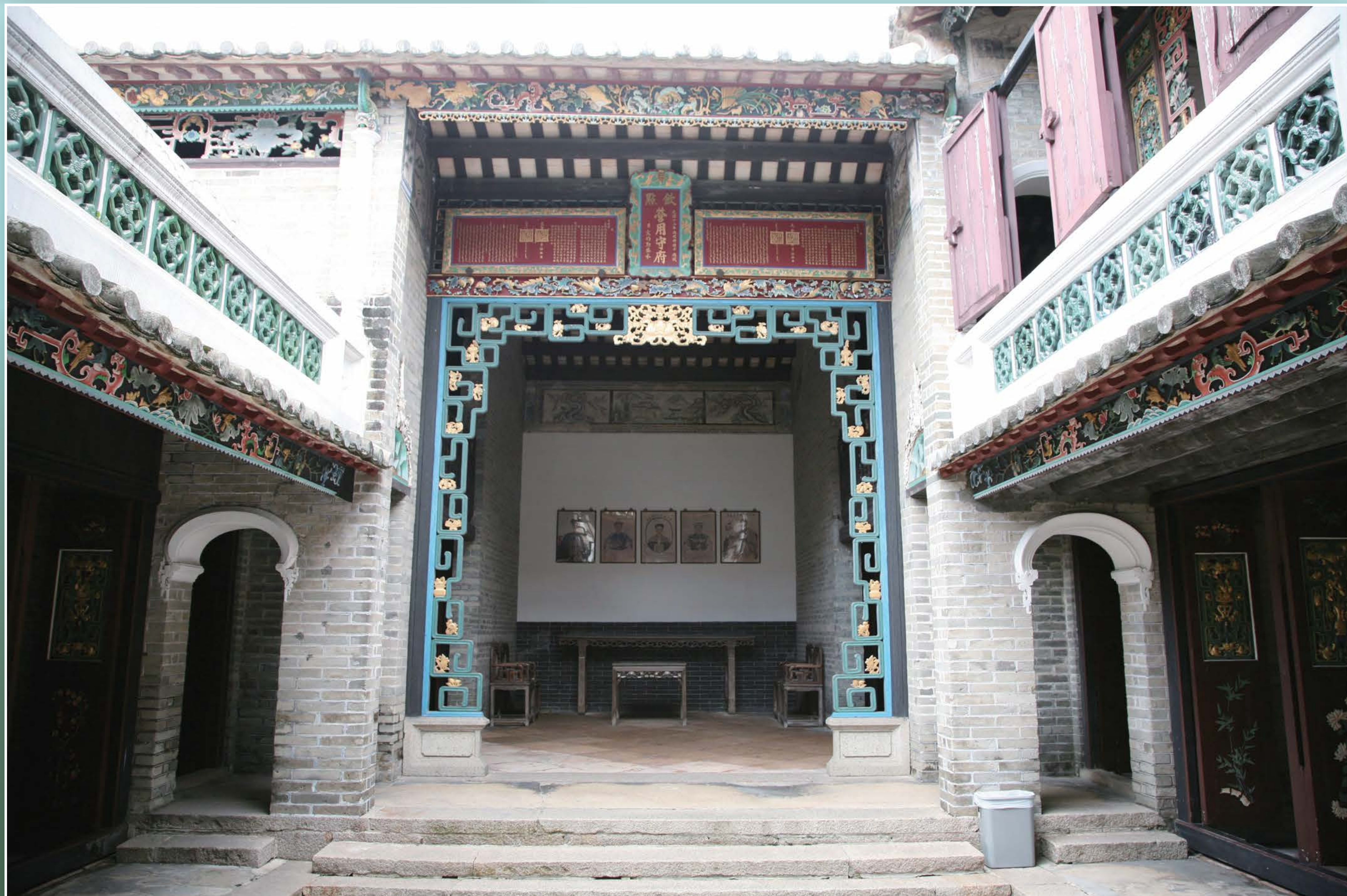
修復後的內貌 Interior view of the buildings after restoration
