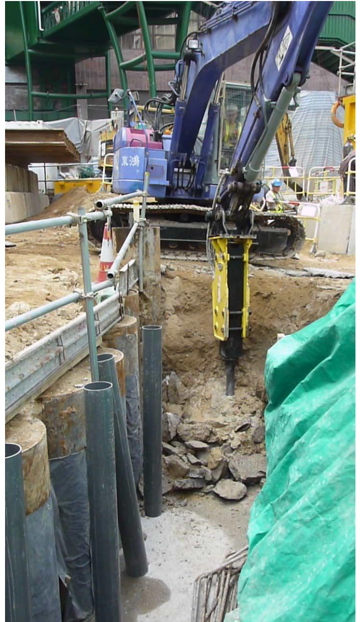
Plate 11.B.18 Photograph showing the drilling of a debris flow boulder to the southwest of the shaft
