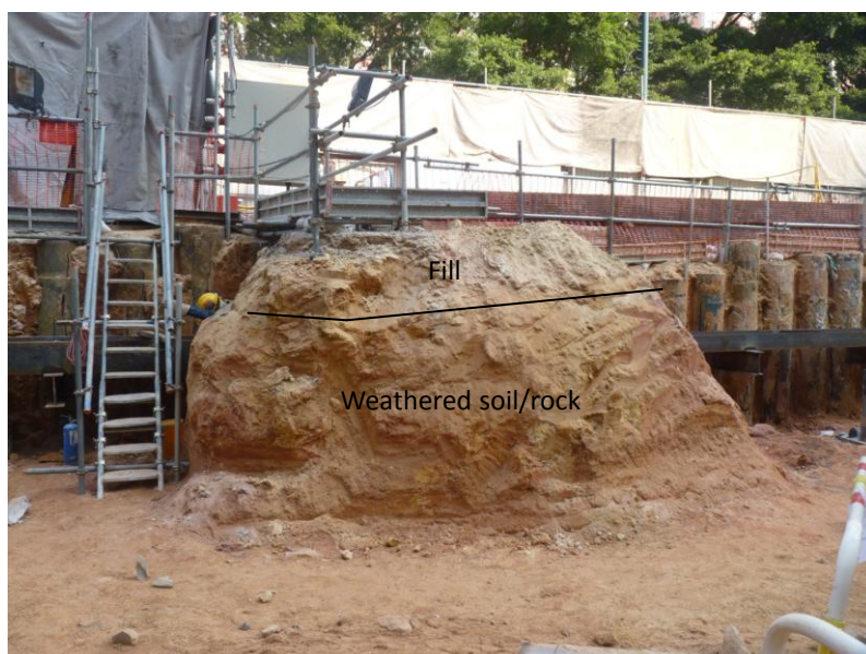
Plate 11.B.1 Photograph taken of the south/centre part of the site, showing the stratigraphy of the site, i.e. shallow artificial fill over weathered soils and rock.
