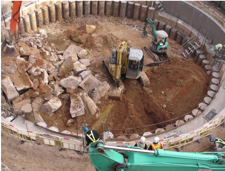
Plate 11.B.7 Photograph showing the eastern shaft excavations in progress; note all the boulders on the left of the photo and the large rock being uncovered.
