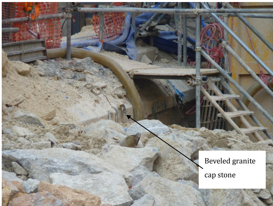
Plate 11.B.4 Photograph showing the top of the retaining wall; notice the beveled granite cap stone.
