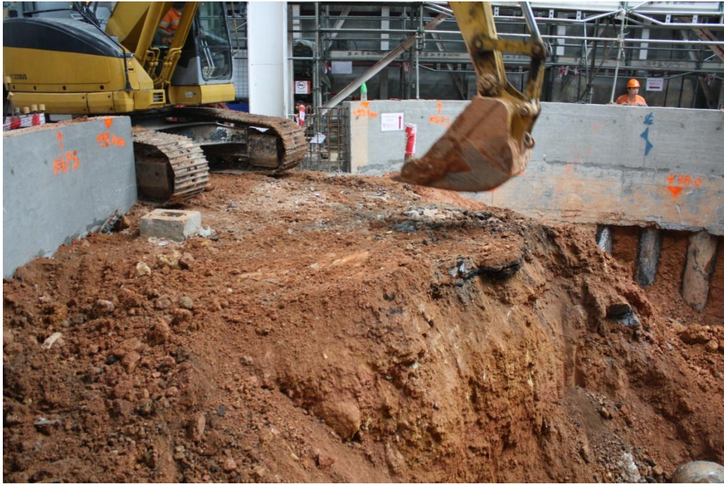
Plate 11.B.37 Photograph of the stratigraphy within the shaft as it is being excavated; view looking west
