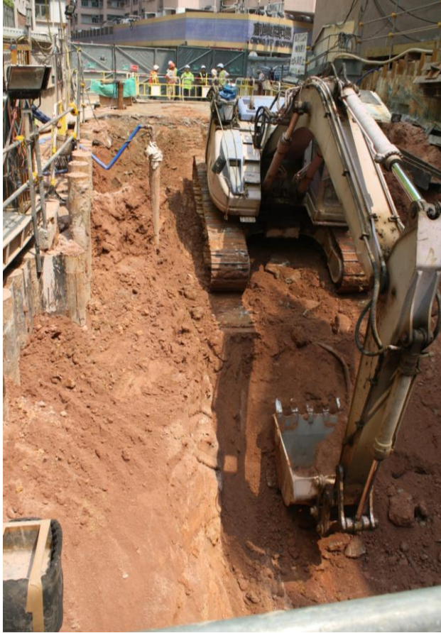
Plate 11.B.15 Photograph showing the area excavated and the deeply weathered red hill slope soils
