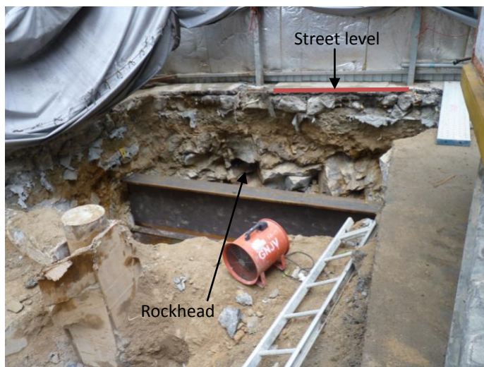
Plate 11.B.6 Photograph showing the proximity of the current surface and rockhead and boulders; notice the cut rock beneath the surface in the centre of the photo. The rock was cut to place the I-beam which carries the working deck
