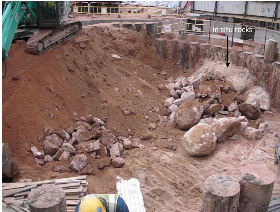
Plate 11.B.9 Photo showing ongoing excavations at the western shaft; note the large rocks appearing to the centre right of the photo at shallow depths
