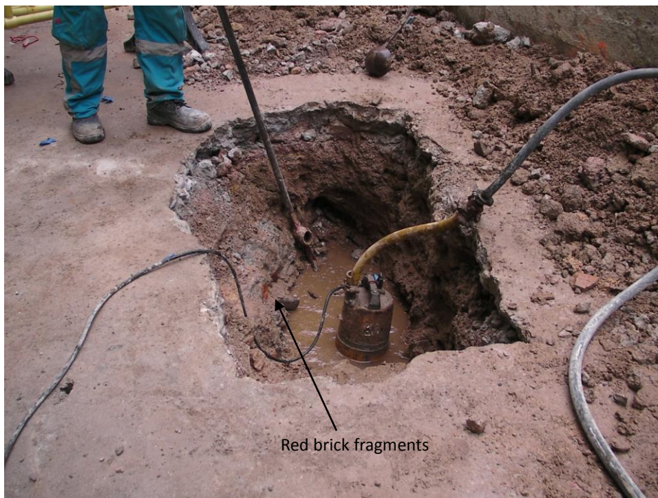
Plate 11.B.14 Photograph showing a view of the utility pit with some red brick visible in the western section and water seepage
