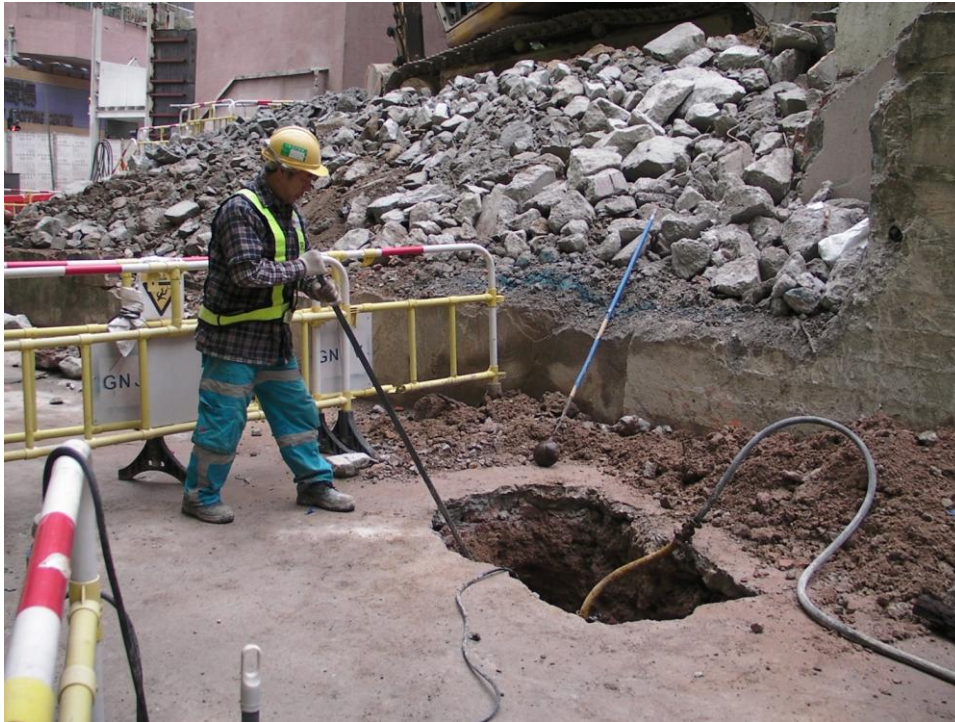
Plate 11.B.13 Photograph showing one of the pits excavated to locate the utilities and a general view north-northeast of the site with the demolition of the public toilets and creation of the artificial ramp needed for piling works
