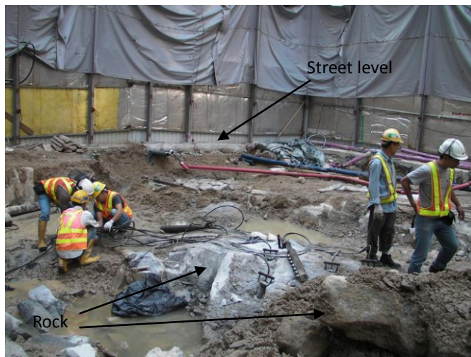
Plate 11.B. 5 Photograph showing large boulders and rockhead at shallow depths; notice the rock in the front right corner and the drilling of rockhead in the centre; the street level is visible in the back of the photo
