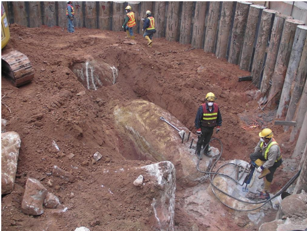
Plate 11.B.8 Rock debris within the eastern shaft at a depth of approx. 2m below the surface.
