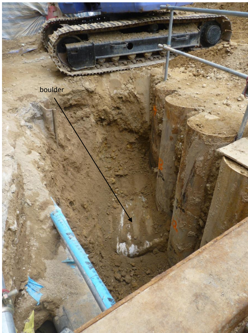
Plate 11.B.19 Photograph showing boulders appearing around 1m below surface set in sterile soils
