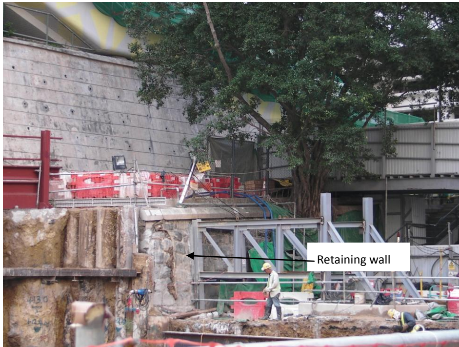
Plate 11.B.3 Photograph showing the retaining wall in the Southwest corner of the works area. The portion will be preserved.
