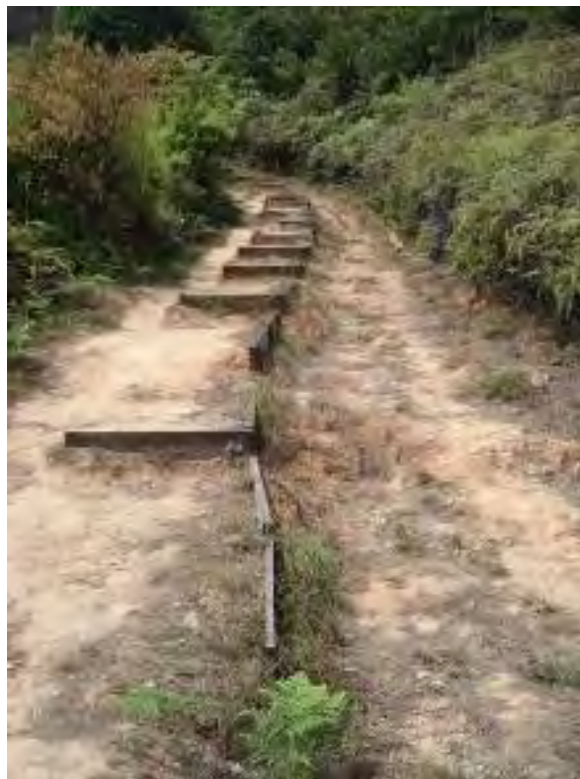
A reworked section with timber boards for reinforcement at Hok Tau Reservoir-Cheung Uk Boulder Trackway
