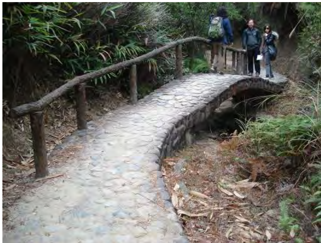
A bridge comprises of stones embedded in the concrete at Tai Lam Chung – Shap Pat Heung Trackway
