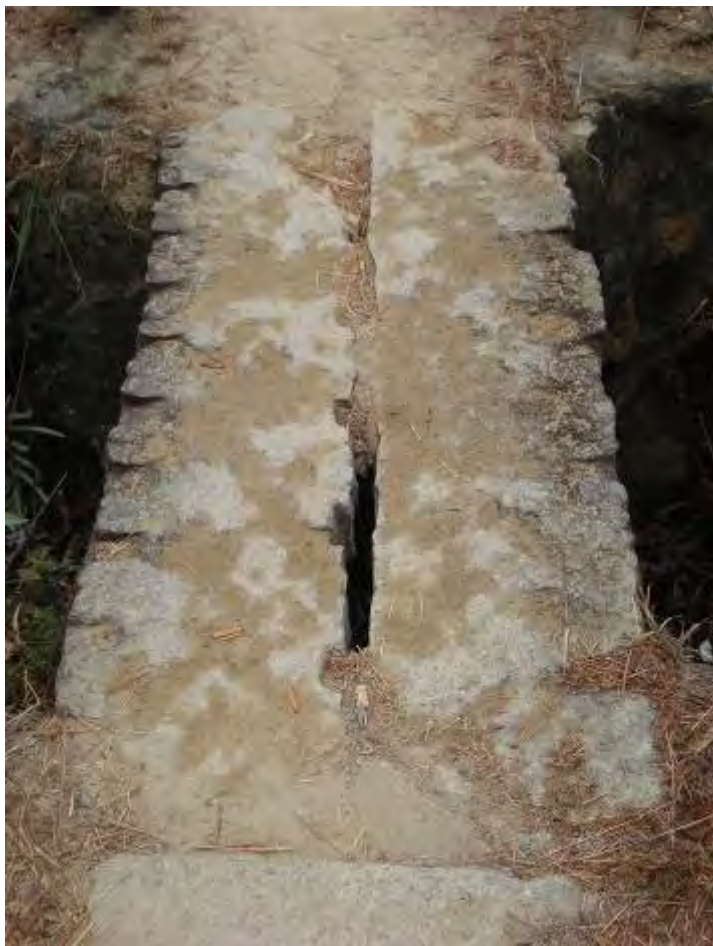
A bridge comprises of feathered granite slabs at Tai Lam Chung – Shap Pat Heung Trackway
