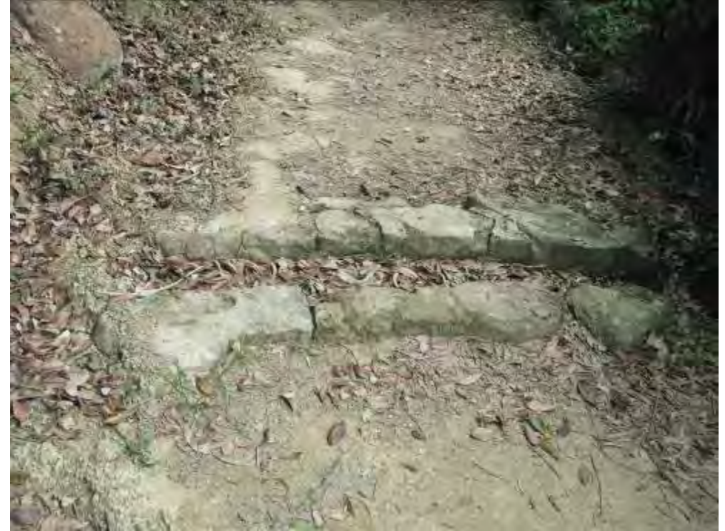
Stone built drains for water diversion and for crossing. Passers-by only need one step to across it at Lau Shui Heung-Kat Tsai Shan Au Trackway
