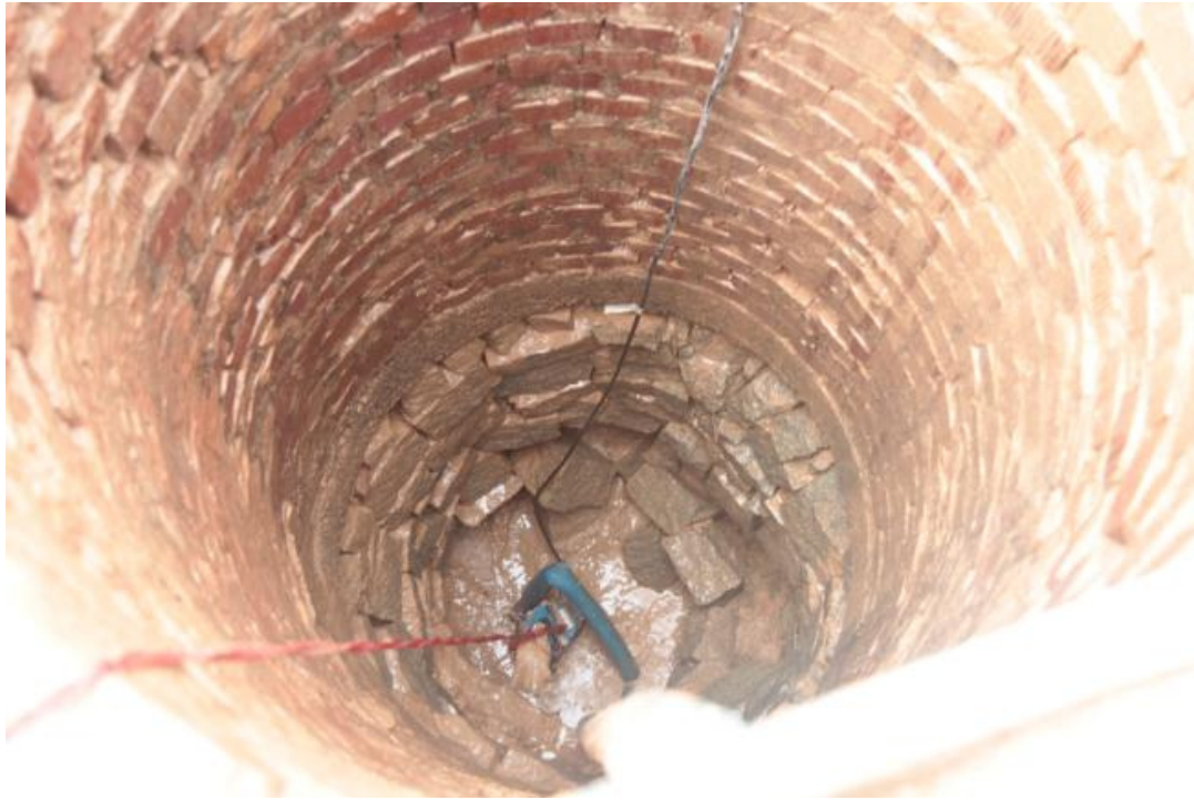
Photo 7: Base of the brick structure.
