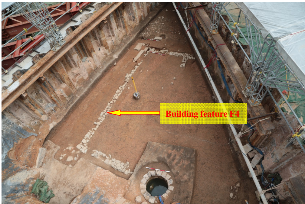
Photo 5: The Song-Yuan building remains were confirmed to be associated with the building structure F4 in Adit C.
