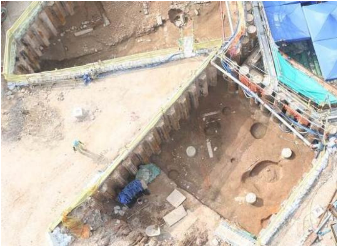
Photo 2: A top shot on Adit C (from northeast to southwest)
