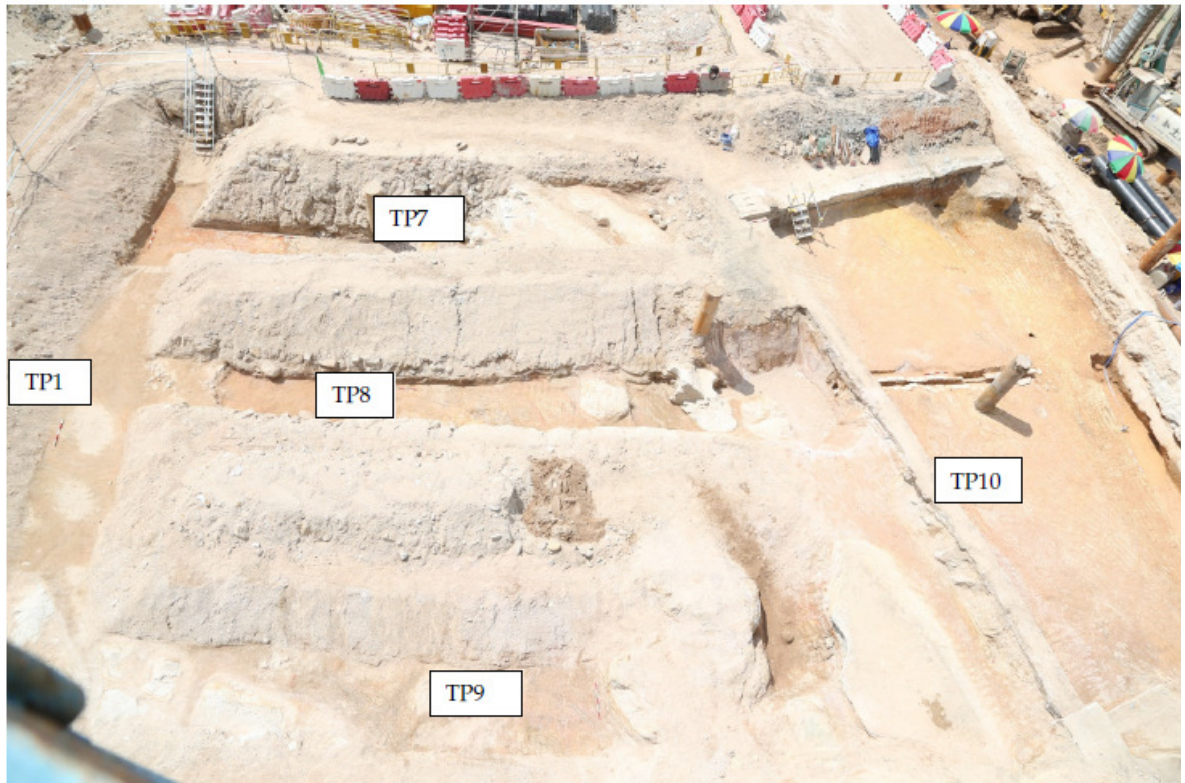
Photo 3: A general view of TP1, TP7-TP10 after excavation
