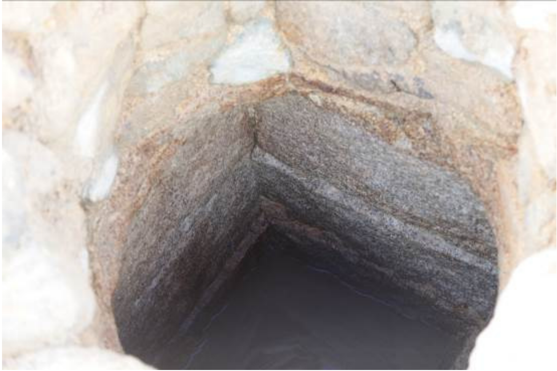
Photo 8: Stone slabs were applied to form a square base.
