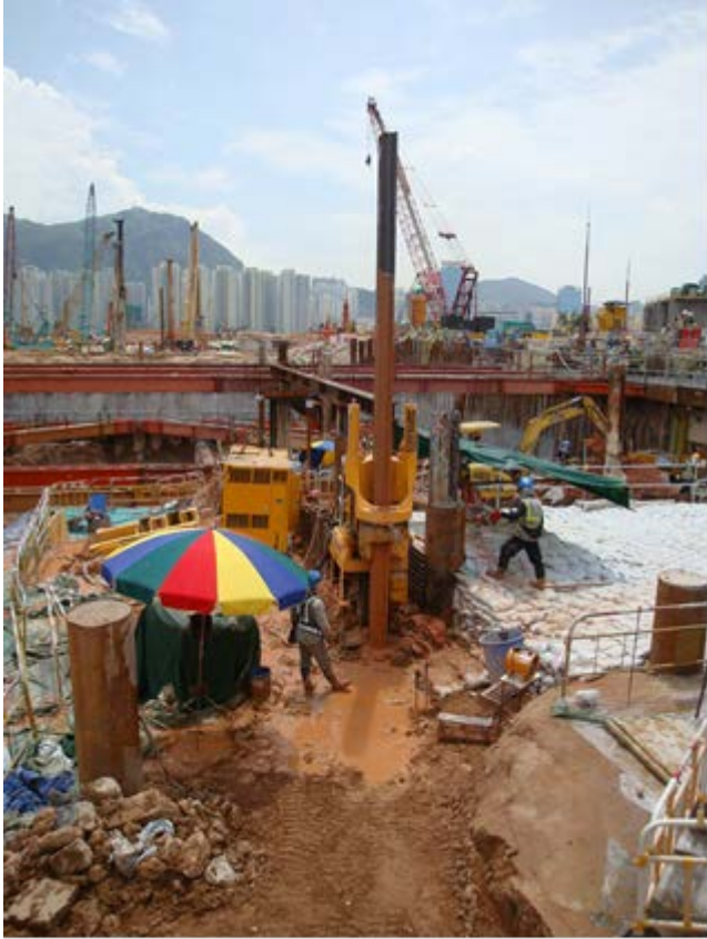
Photo1: Sheet-piling works is being conducted.
