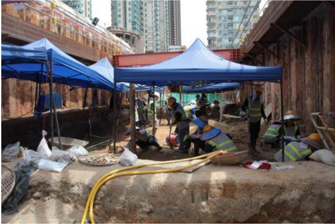
Photo 7: Excavation in Adit C in progress.
