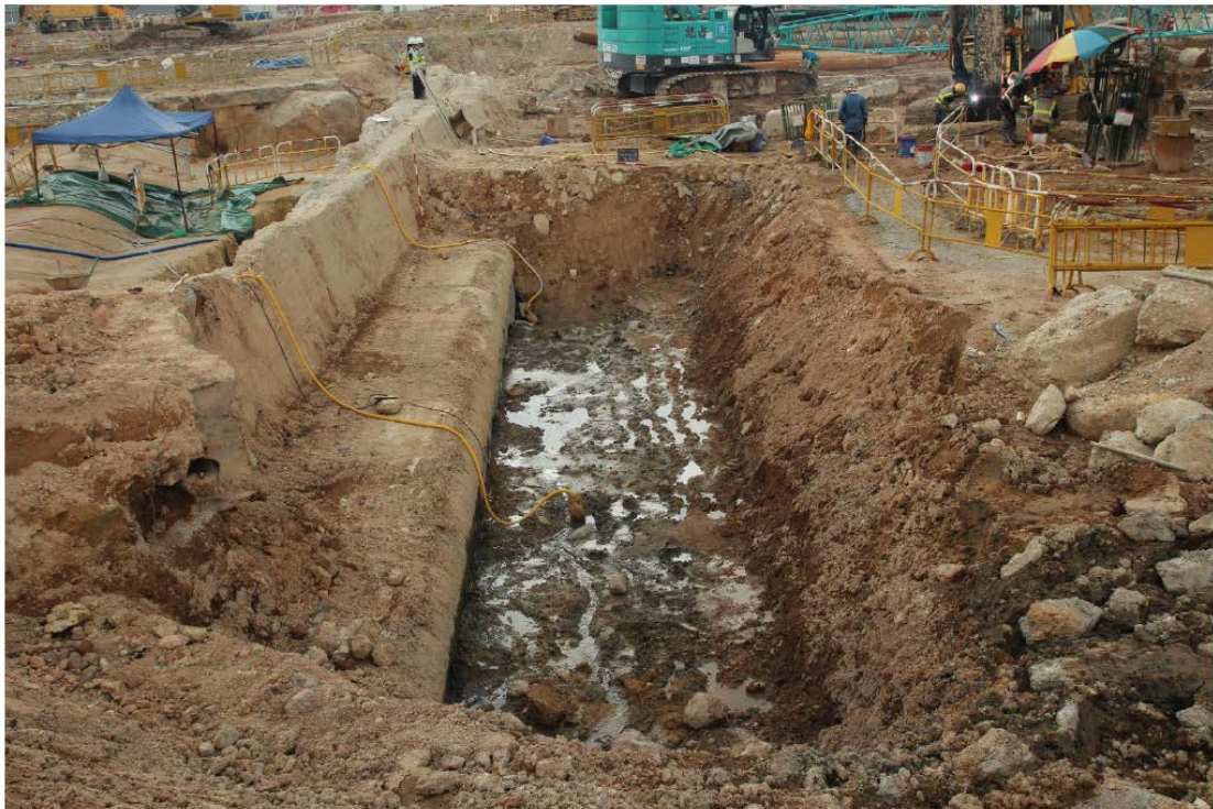
Photo 5: Alignment of the nullah built during the Japanese Occupation.
