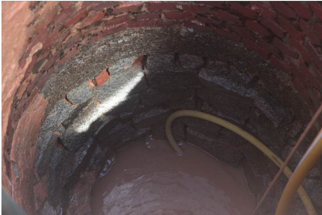
Photo 4: A close up on the lower portion of the structure
