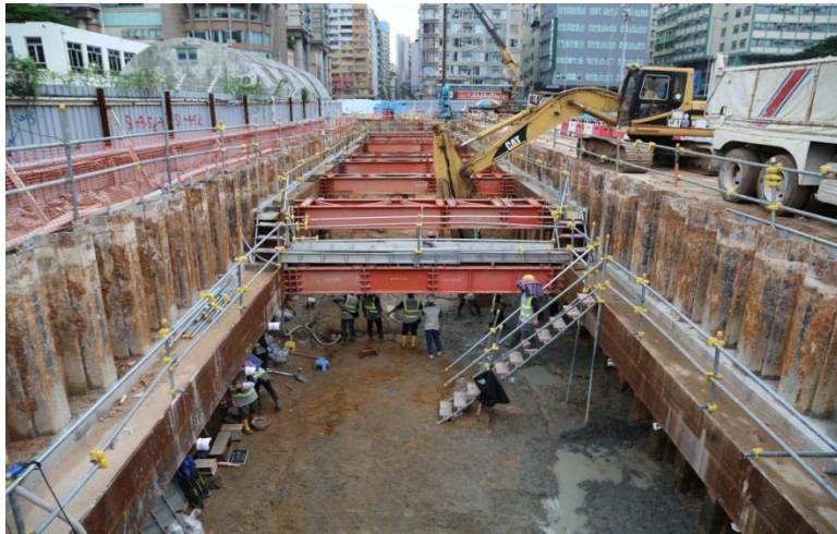
Removing of Fill Layer at Zone C
