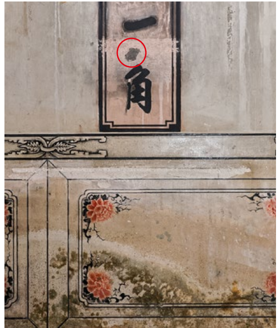
紅圈範圍為適廬內牆身彈痕的修補處，攝於二〇二二年。 The traces of the repair for the bullet strike mark on the wall in Sik Lo, circled red, 2022.
