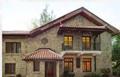
逸夫苑垂脊的彎角末端 The "horned" ends to the hip ridges at the Run Run Shaw Heritage House
