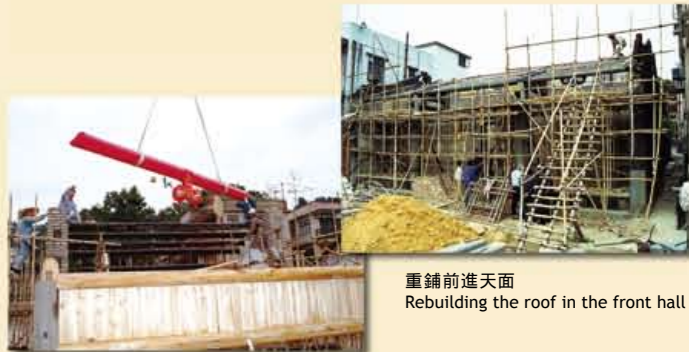
安裝主樑 Installation of the main beam
