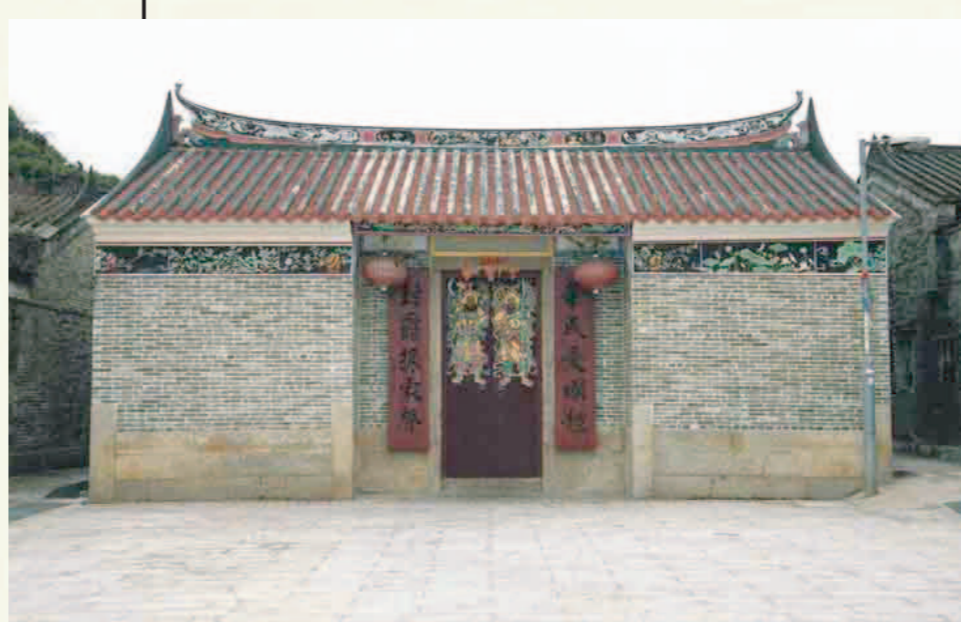
修葺後的外貌 Restored façade of the building
